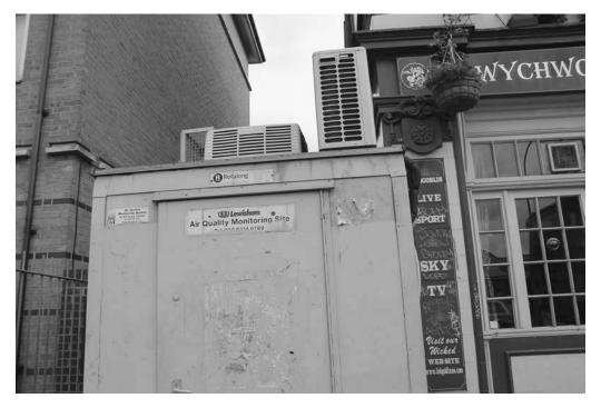
Figure 6.1. London Air Quality Network (LAQN) station. There are over one hundred air quality stations in the LAQN, most of which are managed and run by the King's College Environment Research Group (ERG). Photograph by Citizen Sense.
